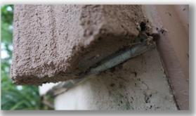
• The stucco has poor clearance from the concrete flatwork. Under current installation standards, there should be at least 1.5 to 2-inches of clearance between the concrete flatwork and the stucco material. There are no visible defects related to this application at this time and **no remedial repairs are recommended.**
