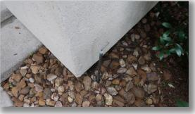
• The lower track / weep screed was observed to be rusted in one or more locations. There are no visible defects related to this condition at this time and no remedial repairs are recommended. The cause of the rust is due to the sprinklers spraying on to the stucco wall.
