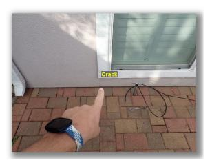
• There is failing and/or missing sealant at and around the window openings. It is recommended to remove and replace all old and failing sealant around the windows to help prevent water intrusion at these locations. It is recommended to use an industry approved NP1 sealant.
