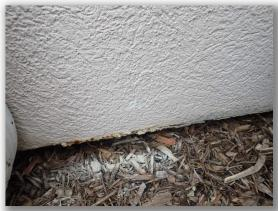
Drill Location E4 Substrate Condition: Compromised Moisture Reading: 20.6
