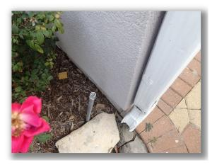
• There is foliage in contact with the exterior stucco finishes. It is recommended to trim the foliage at least 18-inches off the exterior walls.
