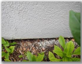
Drill Location F2 Substrate Condition: Compromised Moisture Reading: 14.3%
