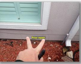
• The area between the exterior cladding / veneer and all of the wall penetrations / openings need to be properly sealed. Areas such as utility connections, downspouts, hose bibbs, lighting fixtures, receptacles etc. It is recommended to use an NP1 sealant.
