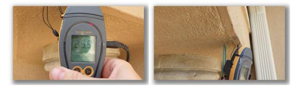
• There is visible bulging and/or releasing of the stucco finish observed. This condition needs to be further evaluated and repairs are recommended.
