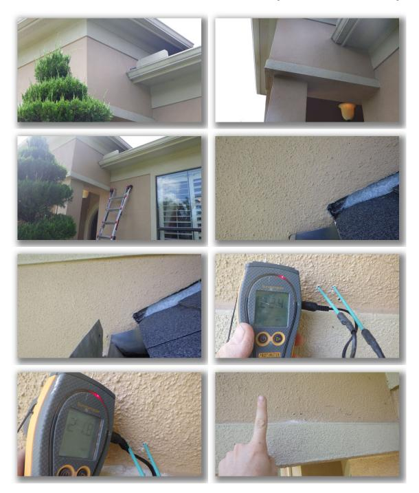
• The ants have built a nest behind the stucco veneer. It is recommended to remove the nest to prevent moisture damage behind the stucco.
